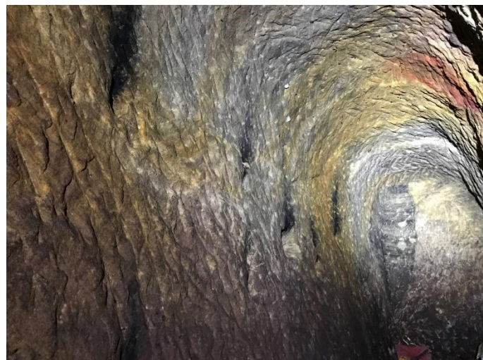
Detail of the adit, with niches for candles along the left hand wall. Note the black carbon staining over each recess from candles which were burning nearly 200 years ago. The shades of yellow and red represent secondary deposits of iron oxide.
