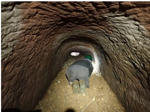
Picture 1. Near the entrance looking out. Note regular pattern of pick-marking on the roof and walls
