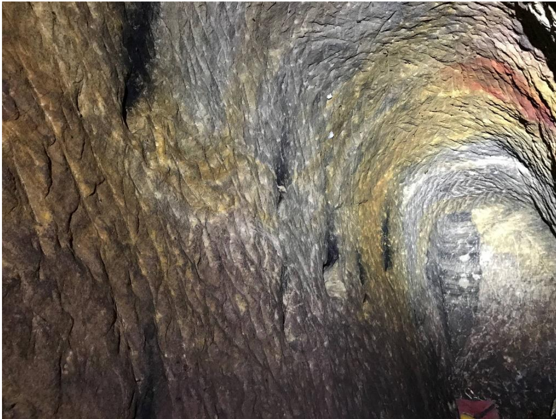
Picture 5. Smaller niches for candles along the left hand wall. Note the black carbon staining from the flame over each recess from candles which were burning nearly 200 years ago.
