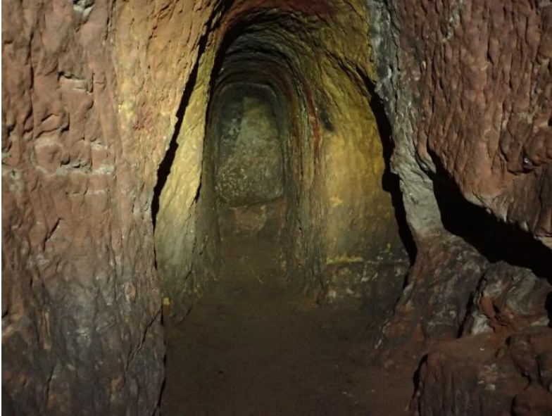
Picture 3. The view towards the tunnel terminus, showing the bench of sandstone left when working finished
