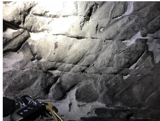
Picture 5 and 6. Tool marks left by a miner using a pickaxe or chisel
